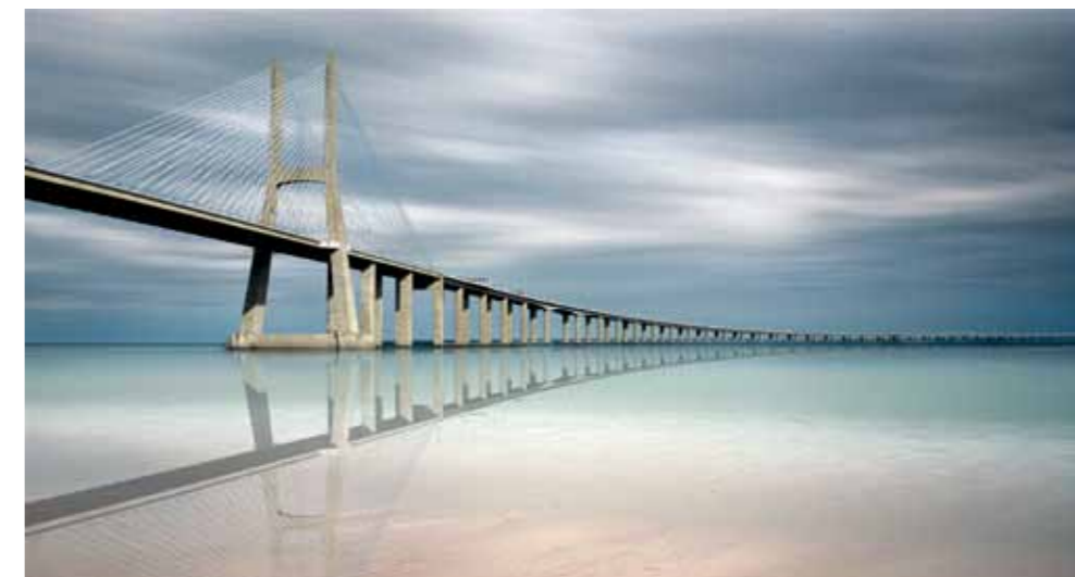
Vasco-da-Gama-Brücke Nicolae Sotir, Frankfurt/Main
